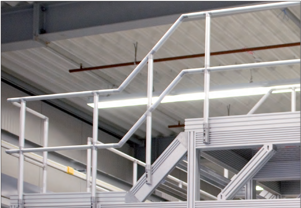
Staircase between two operating platforms.
