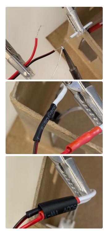
Using a soldering iron, tin the ends of both cables. Then apply heat with the soldering iron to connect them together.
