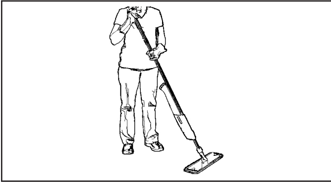
Figure 6. Applying floor finish with Flat Mop (optional).
