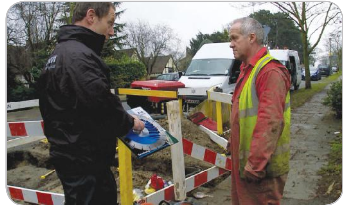
Service & support on site
