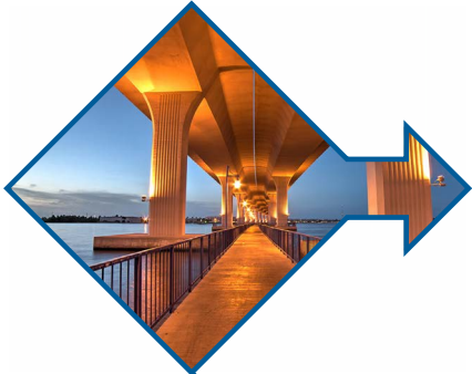
Structural Health Monitoring
