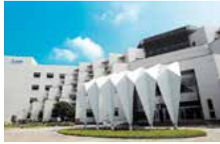
Tainan Plant (Diamond-rated Green Building)
